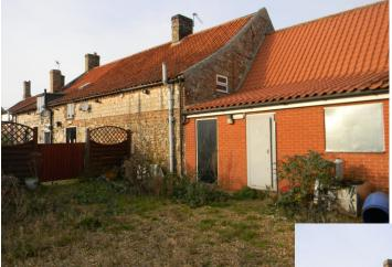
extension from the original property. Where the roof angle changes it matches a thick internal wall location.
